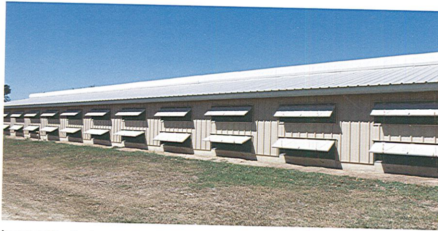
Layer and broiler houses protect birds from the elements. Most houses today, such as this layer house, are well-ventilated and well-insulated and have controlled temperature and automatic lights, feeders, and waterers.
